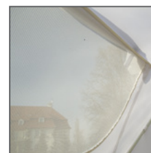
Window holes protected with meshing
